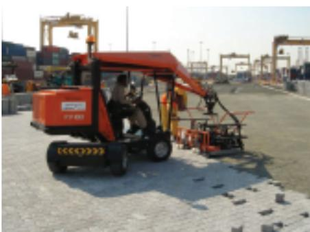
New *Optimas* paving machine model in action
